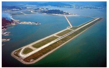
The airport's runway was built on a strip of reclaimed land in the sea, adjacent to Taipa Island, where the main terminal and air traffic control facilities are located. The runway is connected to the apron by two taxiways. The runway length is 3,360m and its orientation is 16/34. Runway 34 is ILS CAT II equipped.
